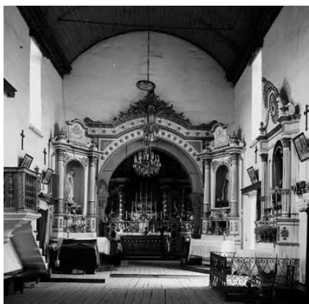
Church. Nave before the intervention carried out by the DGEMN (1968). Source: IHRU archive.
