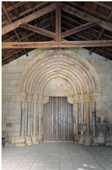
Church, West façade, Galilee, Interior view.
