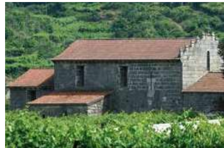
Church. North façade.
