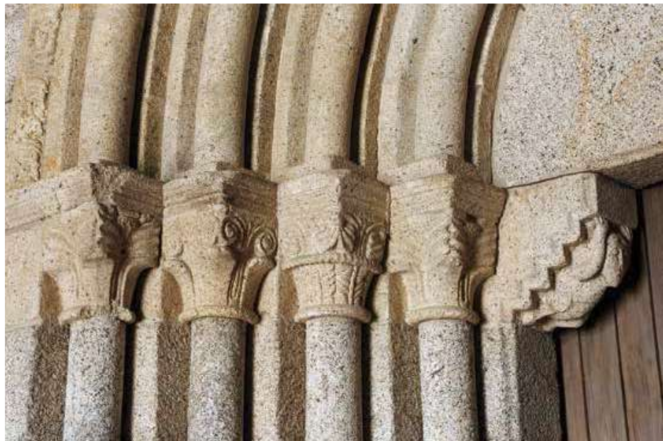
Church. West façade. Portal. Capitals and corbel.
