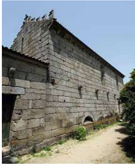
Church. South façade.
