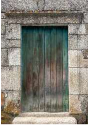
Church. South façade. Nave. Portal.
