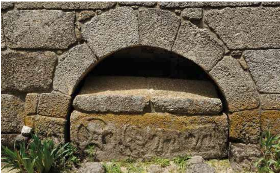
Church. South façade. Nave. Arcosolium.
