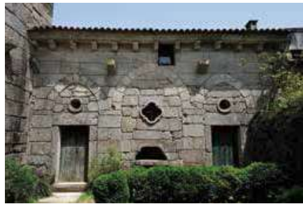
Church. Sacristy. West façade.
