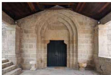
West façade. Galilee and portal.
