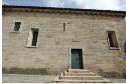
South façade. Nave.
