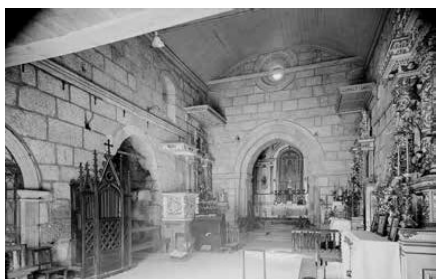
Nave before the intervention carried out by the DGEMN. Source: IHRU archive.
