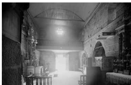
Nave before the intervention carried out by the DGEMN. Source: IHRU archive.
