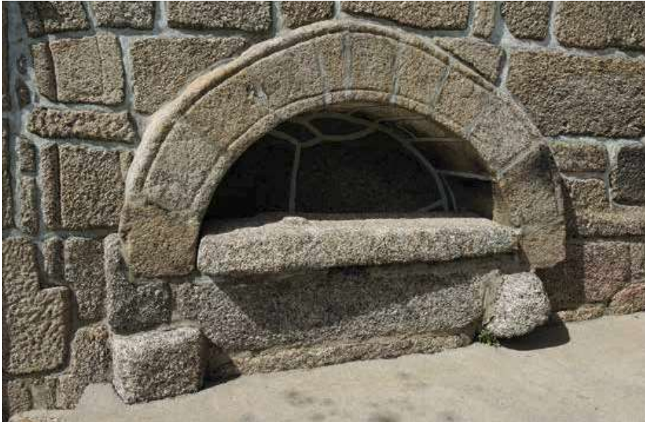
South façade. Nave. Arcosolium. Sarcophagus.
