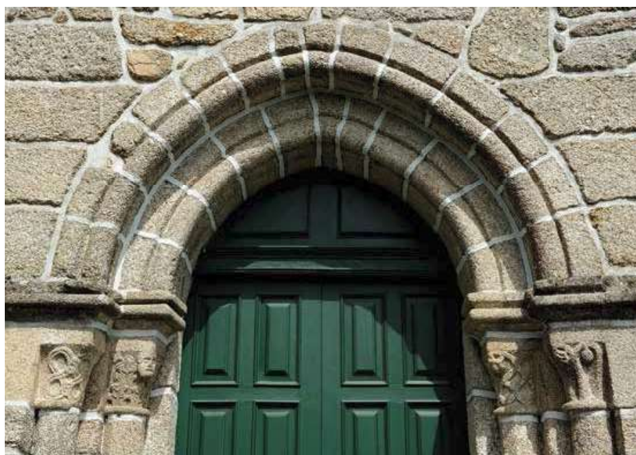
West façade. Portal.
