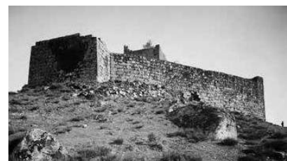
Partial view of the wall before the intervention carried out by the DGEMN. Source: IHRU archive.
