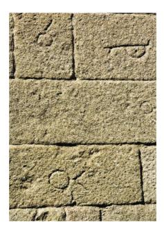
4. Alphabetical and geometrical signs. These masonry markings were used to account for the mason's work. Boelhe's signs, frequent and repeated, suggest that the church was probably made by half a dozen masons.
