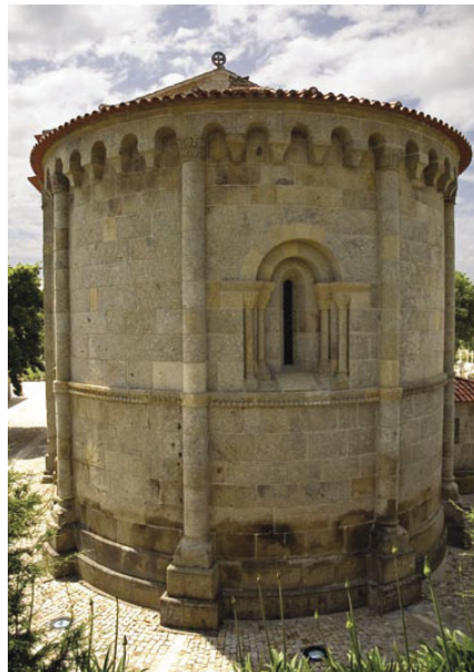
3. The church transept, of semi-circular design, is topped by an arched cornice settled on plain corbels, much like the apsidioles of the Monastery of Saint Mary of Pombeiro and the naves of the Monastery of the Savior of Paço de Sousa.
