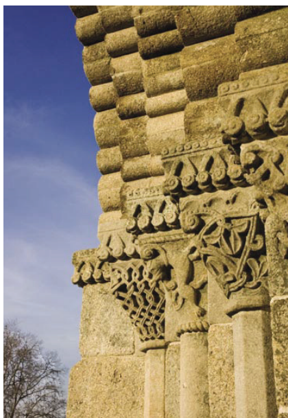
10. West portal. Capitals, lines of ashlars and archivolts.
